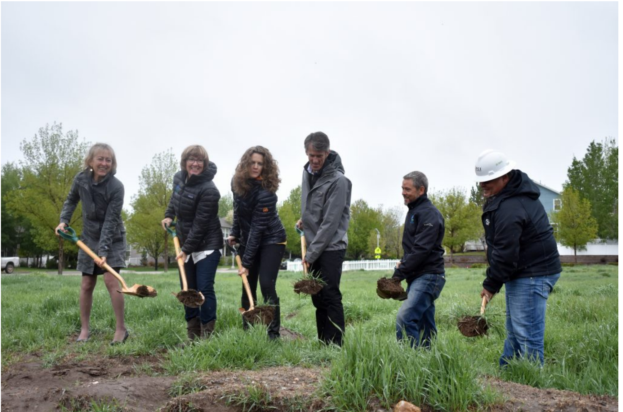
County officials toss some dirt during the official ground-breaking celebration at the Two10 housing project at Eagle Ranch. Shown, left to right, are Eagle County Commissioner Kathy Chandler-Henry, Eagle County Commissioner Jeanne McQueeney, Eagle County Real Estate & Development Manager Tori Franks, JV DeSousa of JV DeSousa LLC Architecture-Planning Eagle County Commissioner Matt Scherr and Gabe Conner General Manger Special Projects Division of FCI Constructors. Special to the Daily by Ken Nager
